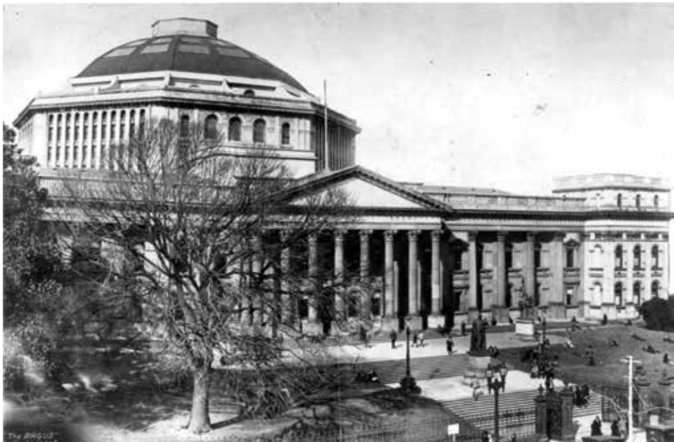
The Library after completion of the reading room. Bates Smart Collection, University of Melbourne Archives.
