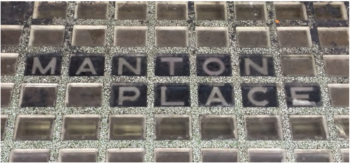
Glass blocks set into footpath at rear of Target store, Little Bourke Street, 2019, photograph by the author
