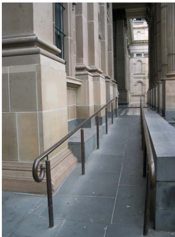
Ramp at front entrance of Library
